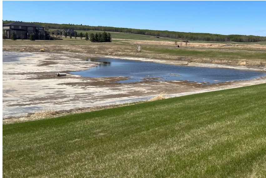
Above: Photo Storm Water Management Area
